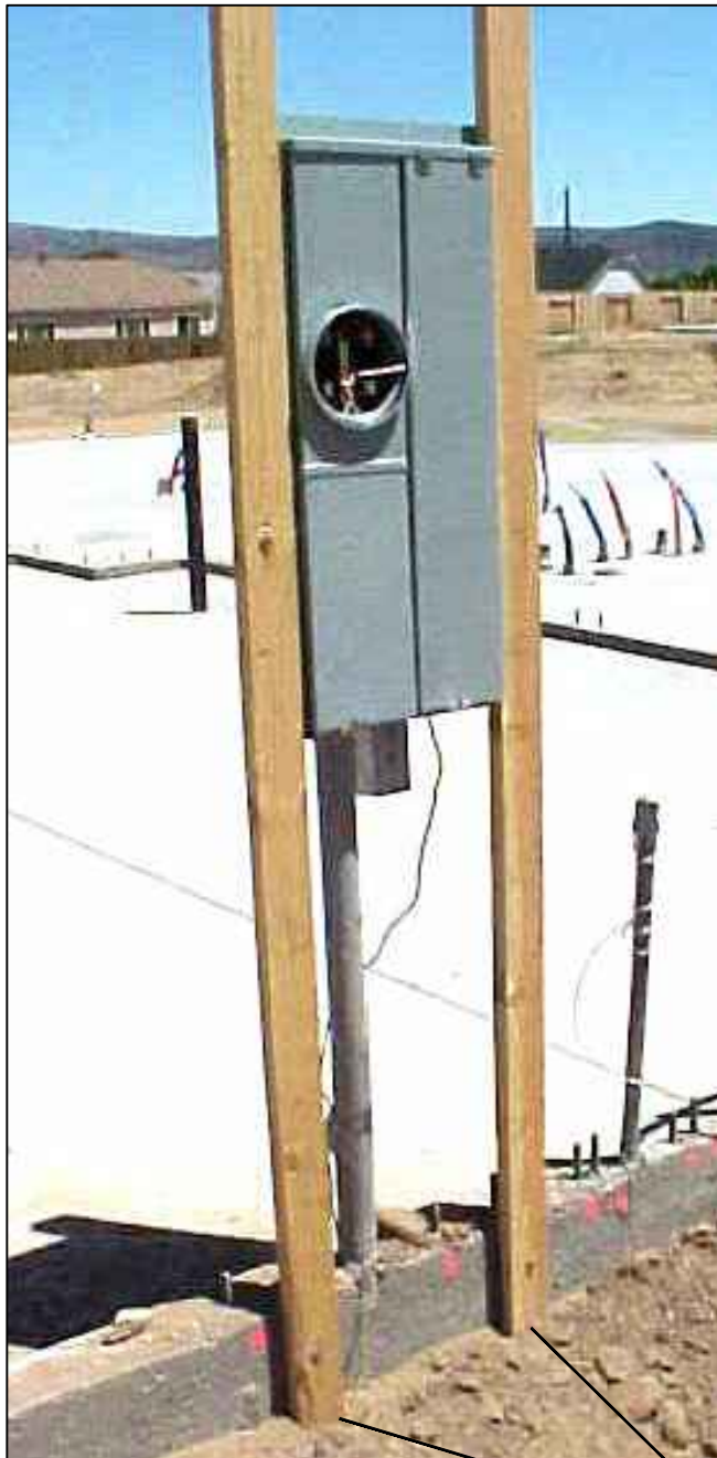
Figure 5 Semiflush Panel Mounting Using 2"x4" Stud Framing
