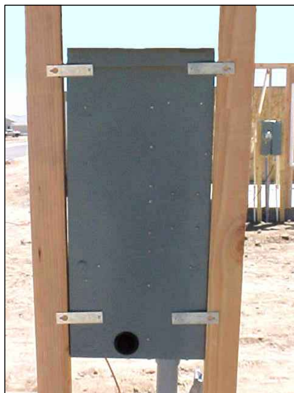
Panel Back Showing Swing Out Mounting Brackets Attached To 2"x4" Stud Framing Figure 4
