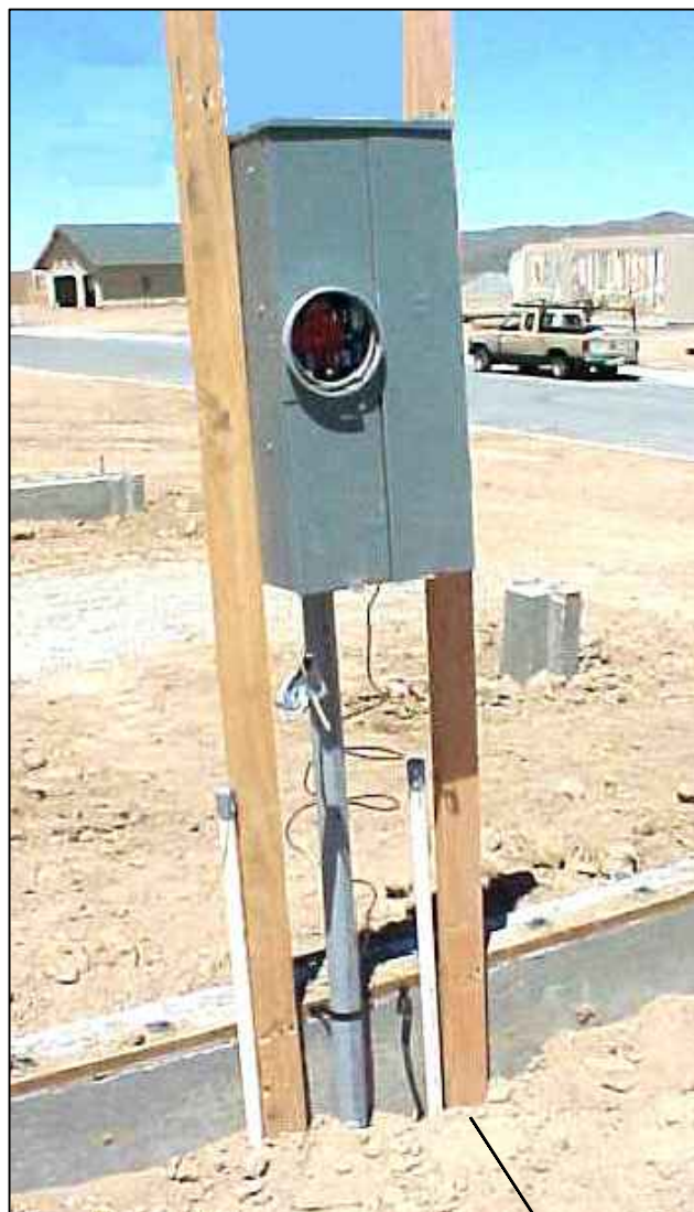
Surface Mount Panel w/ 2"x4" Stud Framing Figure 3
