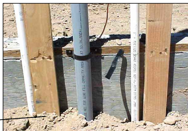
Conduit Support Strap Attached To Sill Plate
